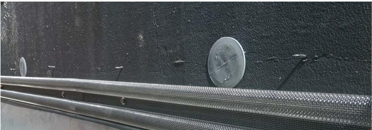
The cavity barriers need to be installed continuously, so if a fire breaks out there is no pathway for the fire to pass.
